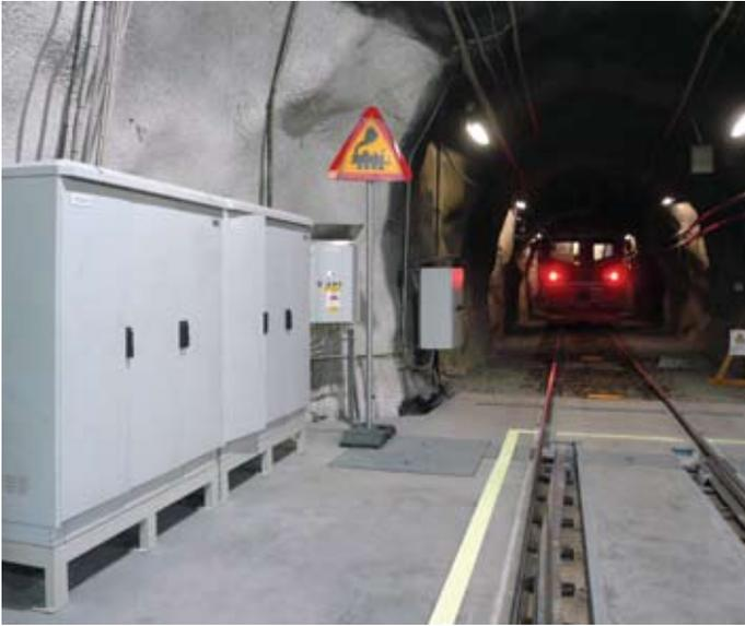
Bombardier's *INTERFLO* 150 solution incorporates moving block technology which allows shorter headways between trains and therefore greater capacity and better utilisation of track space. The solution also comprises a purpose-designed control system and onboard equipment for nine production locomotives and up to five service and maintenance vehicles.
